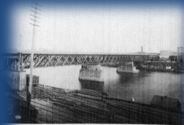
PENNSYLVANIA RAILROAD COMPANY'S BRIDGE OVER SCHUYLKILL RIVER ON FIFTEENTH STREET (LATER RAILROAD) PHILADELPHIA
